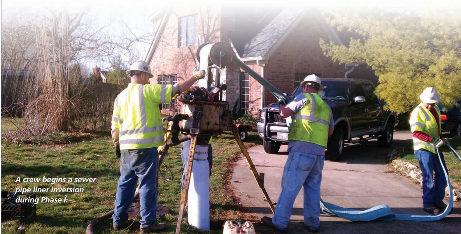
**A crew begins a sewer pipe liner inversion during Phase I.**
