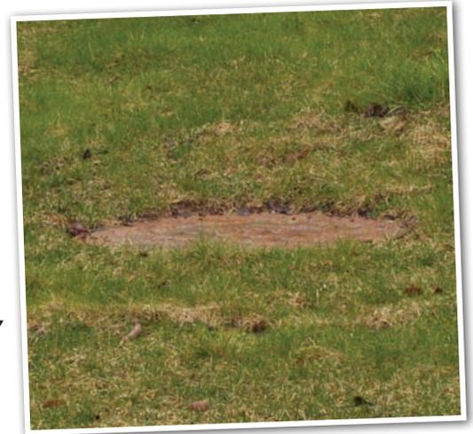
**This manhole was found in a yard during a maintenance check buried under 2" to 4" inches of dirt and sod. Our crew uncovered and raised it to grade.**
