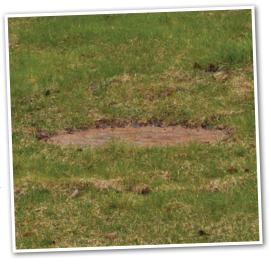
This manhole was found in a yard during a maintenance check buried under 2" to 4" inches of dirt and sod. Our crew uncovered and raised it to grade.
