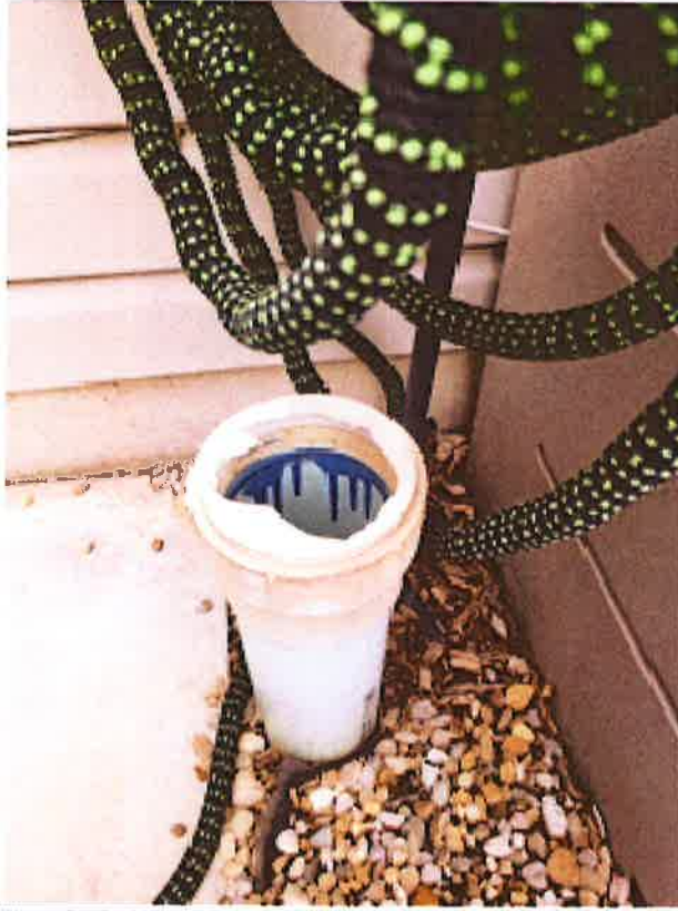
Photo Examples of Broken/Missing Cleanout Caps:
