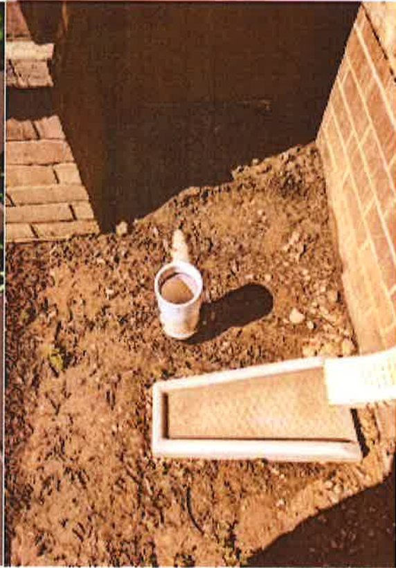
Photo Examples of Broken/Missing Cleanout Caps:
