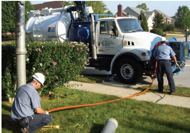
Bobby Patton and Dan Raley carefully perform the line cleaning operation in the Timber Bend neighborhood utilizing the District's GapVax truck.
